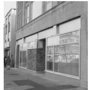
Restored façade adding to streetscape
